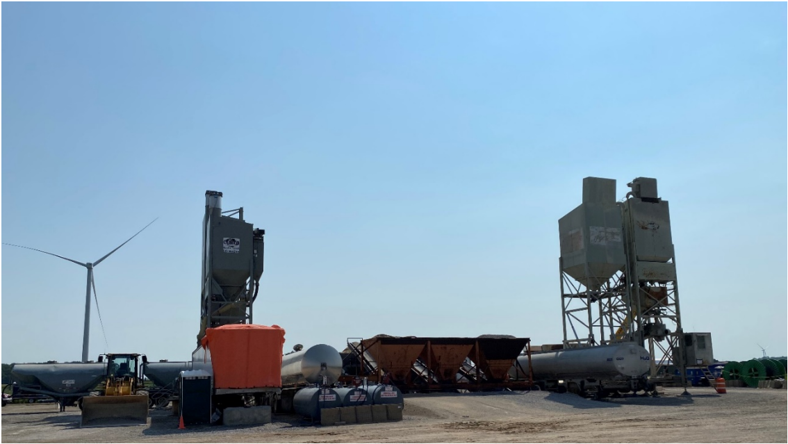
Figure 2-3 Steel concrete mixing structures with material hoppers, water trucks and fuel tanks
