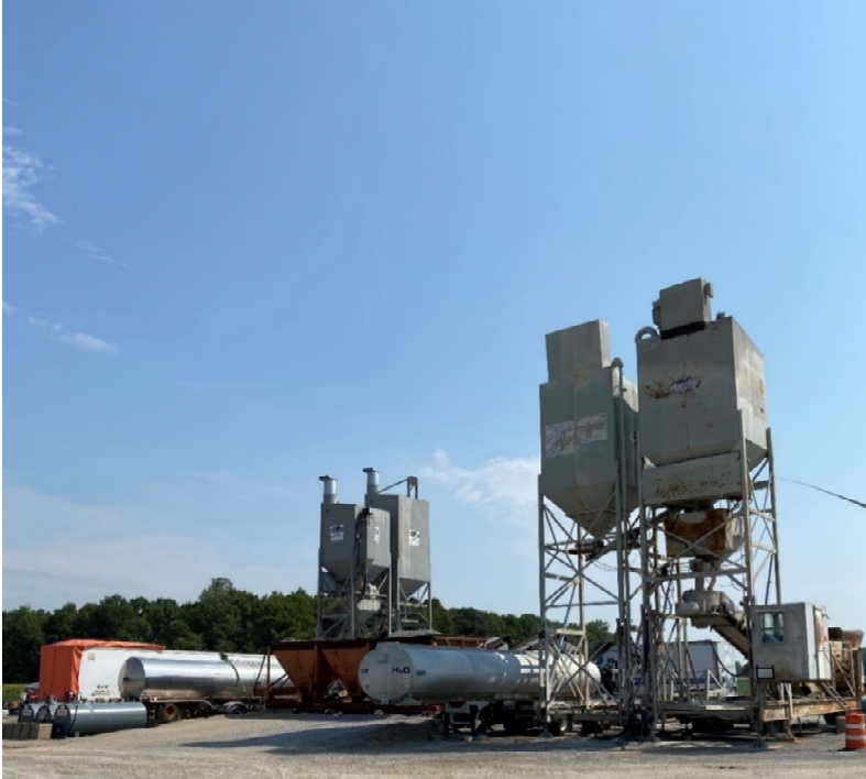
Figure 2-2 Steel concrete mixing structures and water tanks
